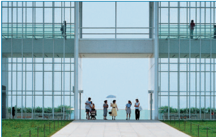
Tokyo Kasai Rinkai Park View Visitors Center Chiba Prefecture, Japan (Complete project details on our web site)
