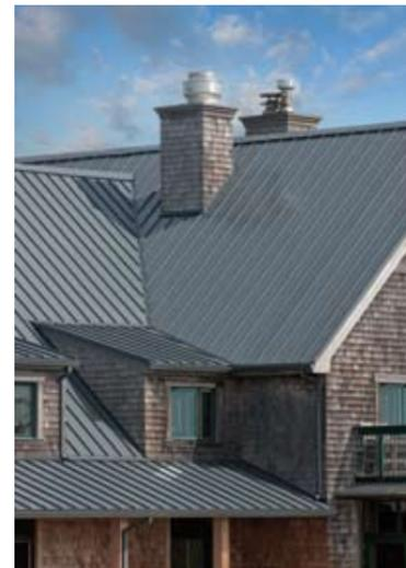
Pacific Gas & Electric, a California utility, found that substituting high-reflectance roof coatings in place of low-reflectance products generated energy cost savings of up to \$2.18 per square foot of roof area.
